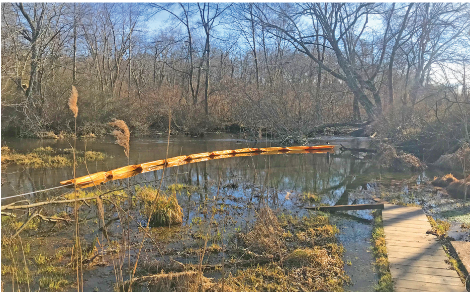
The river right below the Lily Lake dam. A pump connected to heavy machinery snaked along this pathway in November, and now a turbidity curtain is here. MT/Waszyński
